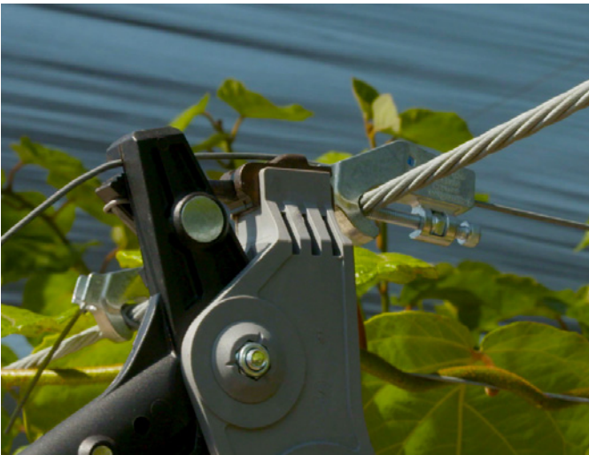
GP90 - Tensioning using Gripple Torq Tool.
