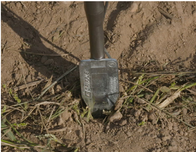
APEX anchor being driven into the ground.
