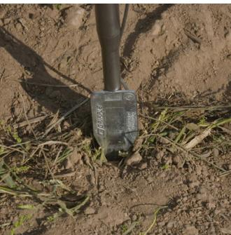
APEX anchor being driven into the ground.
